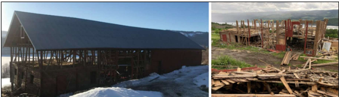
Photo 3.1-1 Barn structure in Brøttum, Ringsaker and its dismantling process [13]
